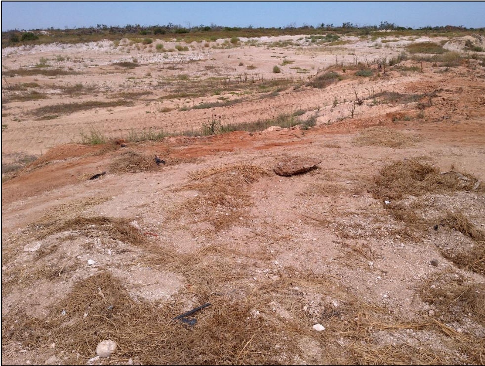
Figure 53. View of the existing borrow pit situated on the western boundary of the proposed Borrow Pit 22 (BP22).
