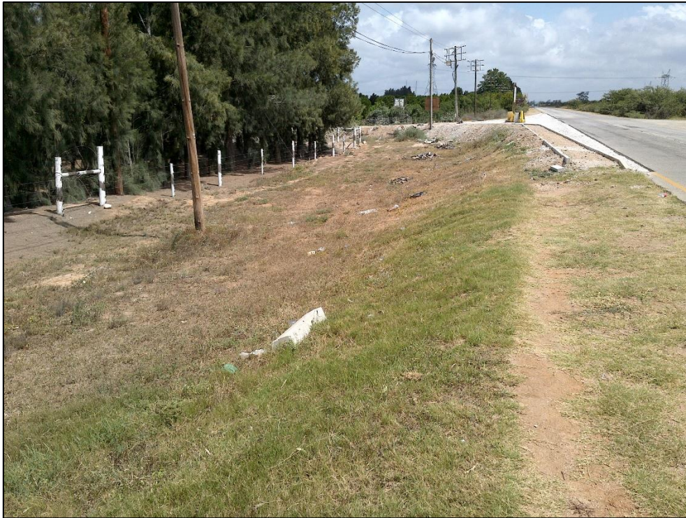
Figure 11. View of the road reserve proposed for upgrade (km 0.5 – km 12) facing south towards Addo Town showing the recent construction of a pedestrian walkway / pavement into the Main Street leading to Nomathamsanqa Township.
