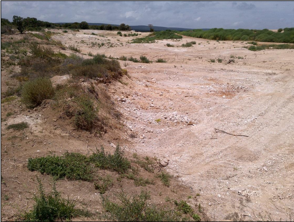
Figure 48. View of the existing borrow pit situated on the southern boundary of the proposed Borrow Pit 20 (BP20).
