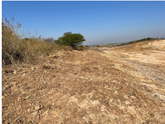
Figure 4 – Cut and fill activities on site
