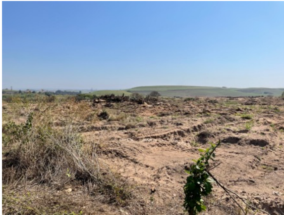
Figure 3 – Vegetation clearing on site
