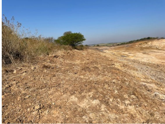
Figure 4 – Cut and fill activities on site
