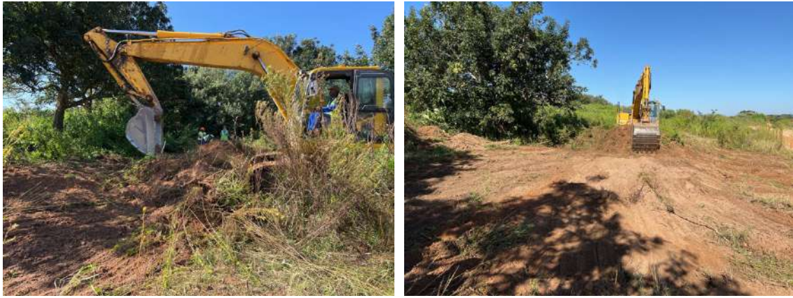
Figure 14 – Mechanical removal of material
