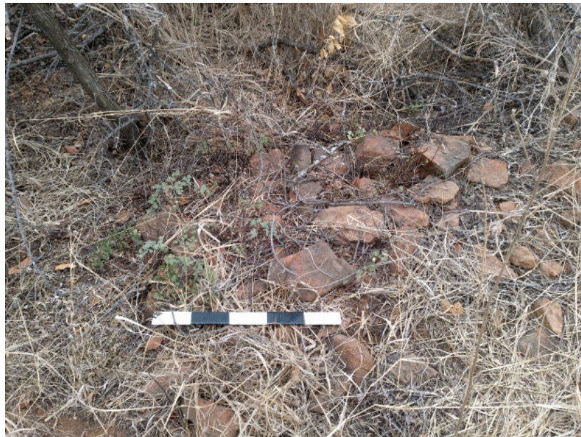
Figure 9 - Collapsed walling feature
