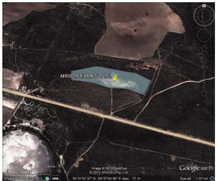
Figure 6: Aerial view of existing borrow pit at km 46.65 (Google earth image, April 2012)
