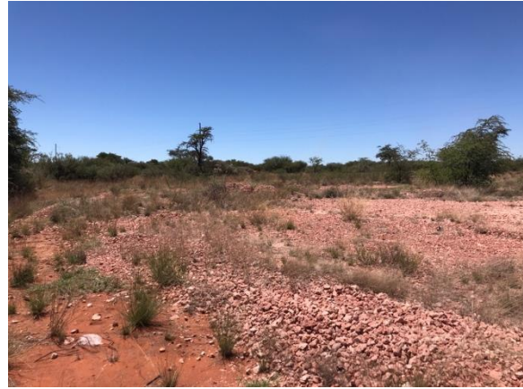
Figure 15: View of graded calcrete gravels within and adjacent to the Gamagara borrow pit.
