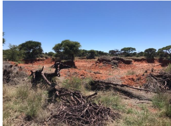
Figure 7: Vegetation clearing within the Woon borrow pit.
