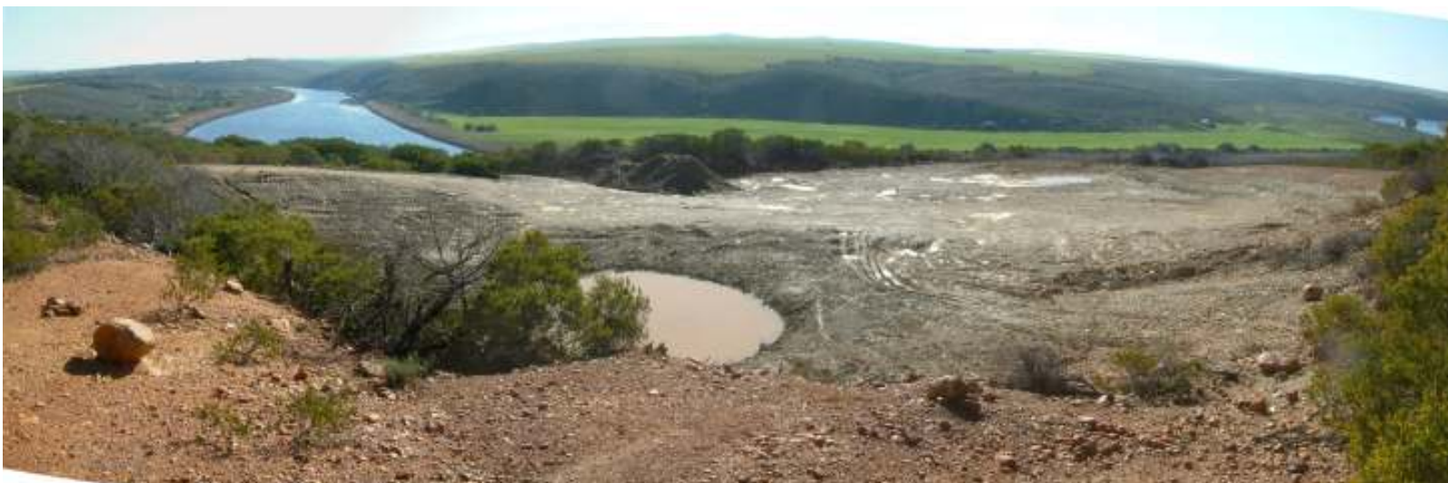
Figure 5: Panoramic view of the existing pit at MR00268/46.8 taken from approach track, with the Breede River in the background sampled stockpile of ripped shale gravel in centre far-foreground (June 2011)
