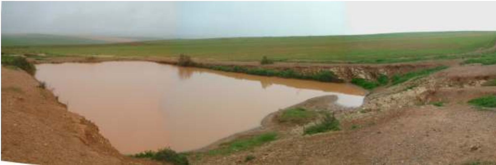
Figure 4: At km 9.0 (8.6) view of easternmost, water-filled, existing pit and surrounds (June 2011)
