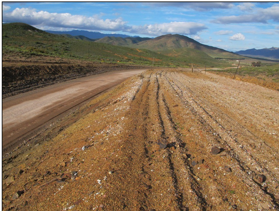
Figure 5: View along the partly-rehabilitated affected area towards the east. The unfenced slope at the eastern end lies beyond the bend in the road.
