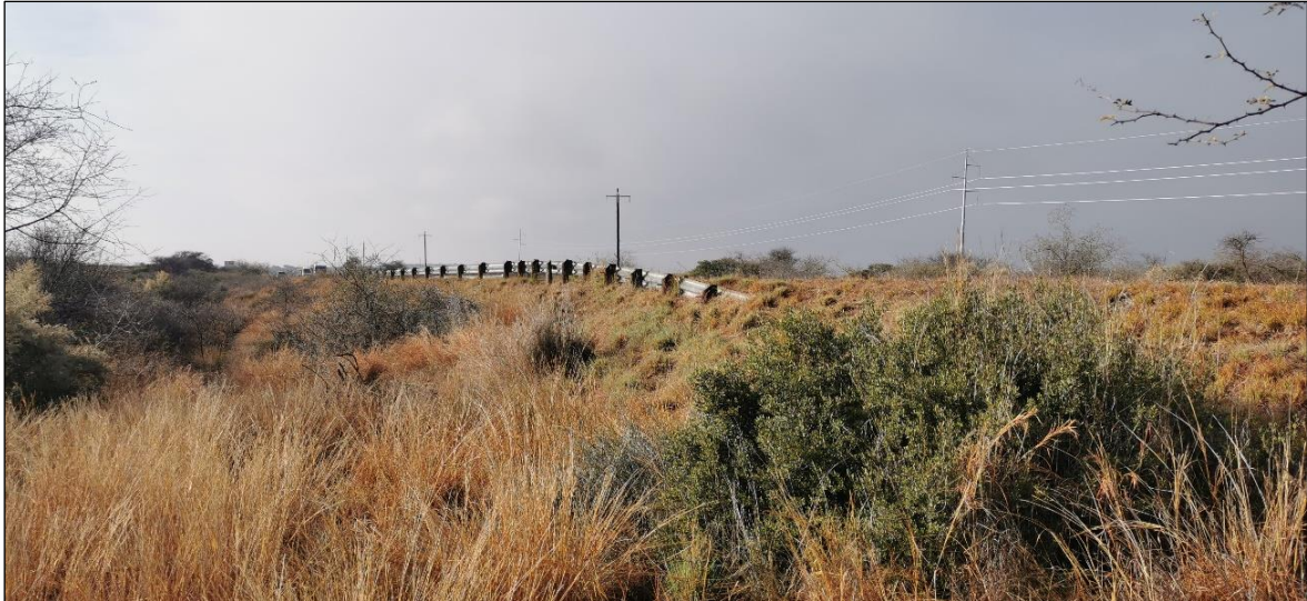
Figure 6 - View of existing powerlines in the area, along the R31 main road.
