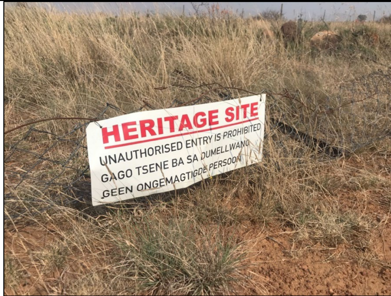
Figure 37: The fence demarcating the site needs repair.
