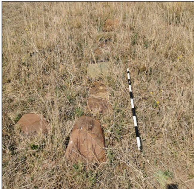
Figure 33: View of the foundation at LDS-01.
