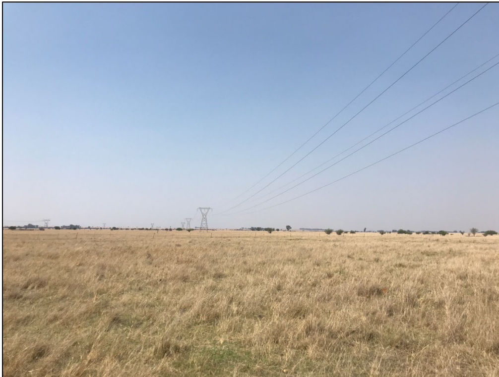
Figure 13: View of existing powerlines.
