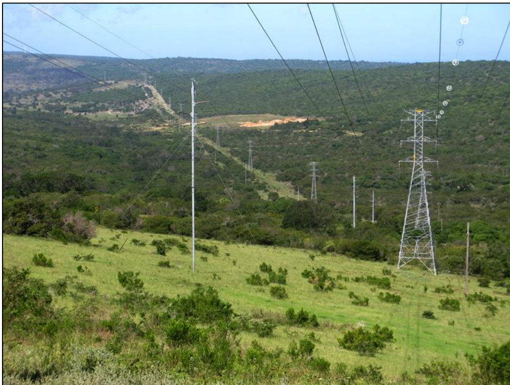
Figure 5. View south-westwards along existing powerline towards sand mine NE of Lemoenfontein showing hilly terrain east of the Gamtoos River Valley.
