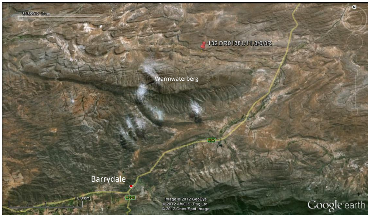
Figure 1: Google earth image showing the location of the proposed extension of an existing borrow pit DR1381/11.3/0.3R (Vidamemoria pit no.132). The relevant 1:50 000 topographical map is 3320DB Plathuis.
