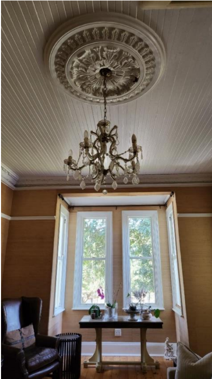
Over elaborate ceiling rose and cornices added to existing drawing room and dining room.
