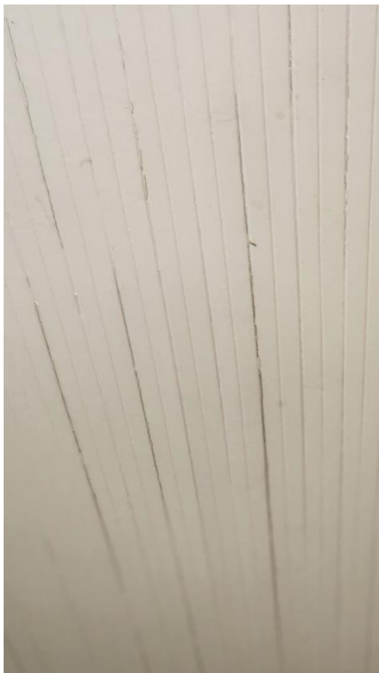
The original ceilings are sagging and rotten in many places.
