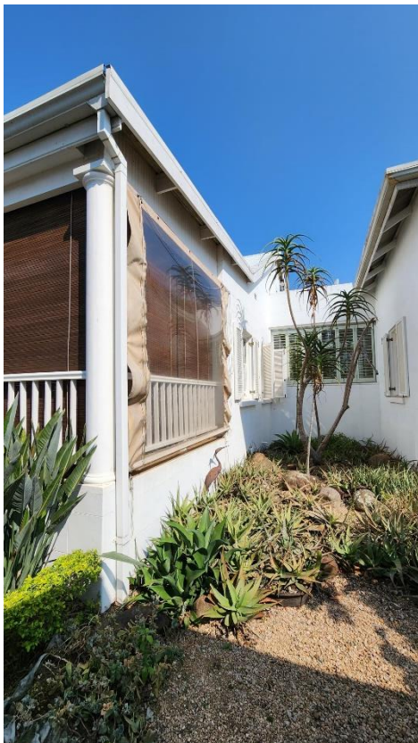
The view of the link from the north.
