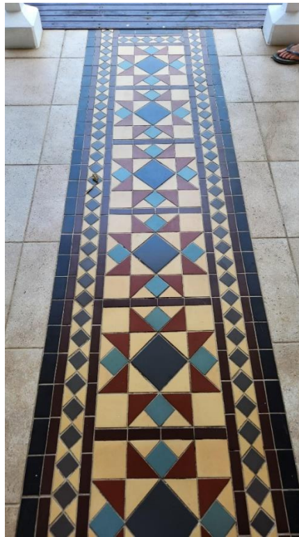
'Runner' of encaustic tiles to new front door.
