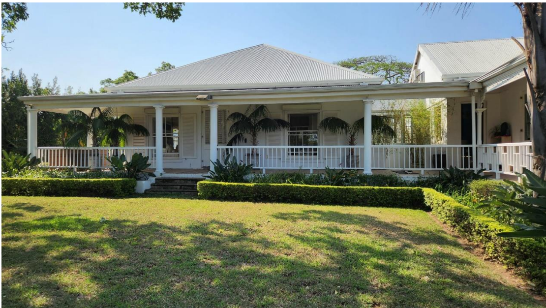
Two bedroom extension added in 2003. The addition was separated from the original house by a link. The veranda has Tuscan Doric columns to indicate intervention.
