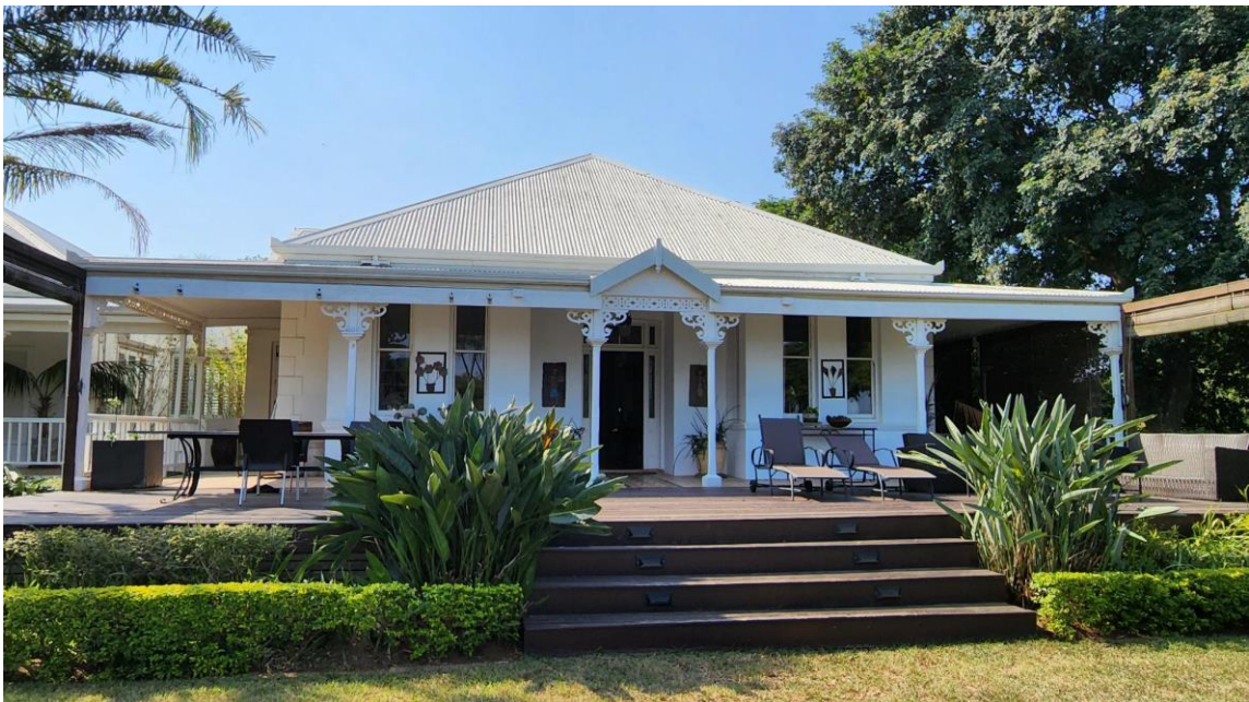
The south facing original veranda. The balustrade was removed as the veranda was extended with decking.
