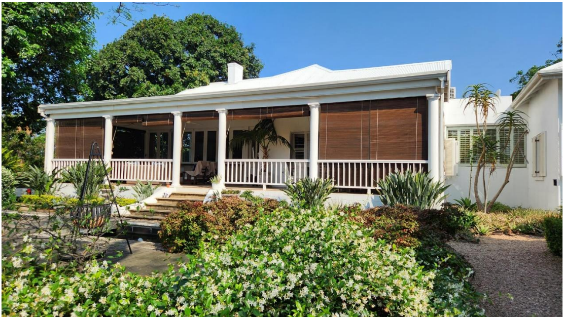
North facing veranda added to the rear of the house to create a new entrance 2003.
