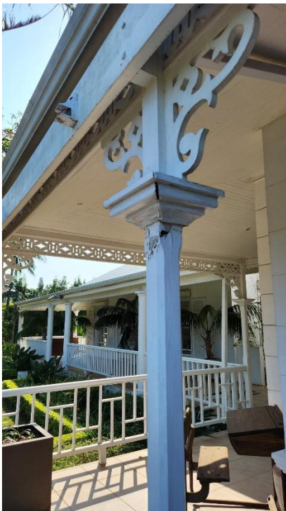
Rotten posts and balustrading requiring repair.
