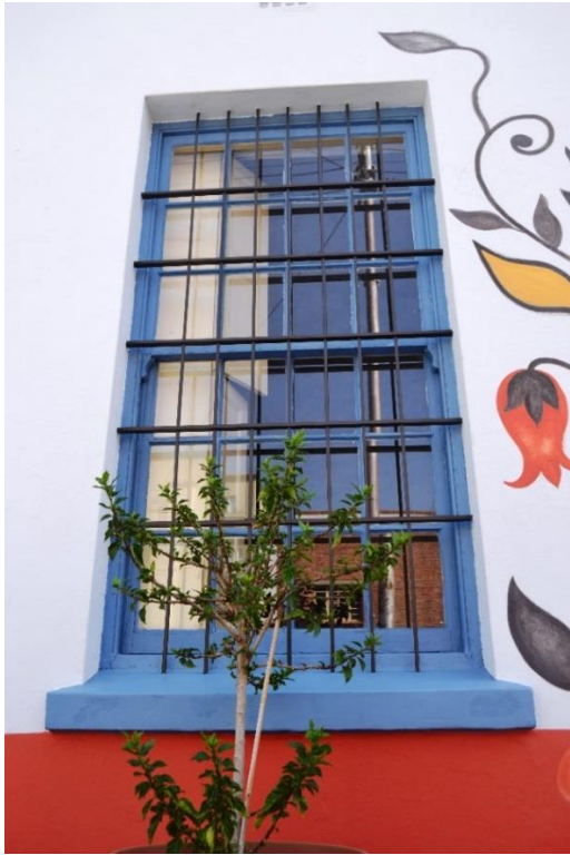
Window on Rose Street facade
