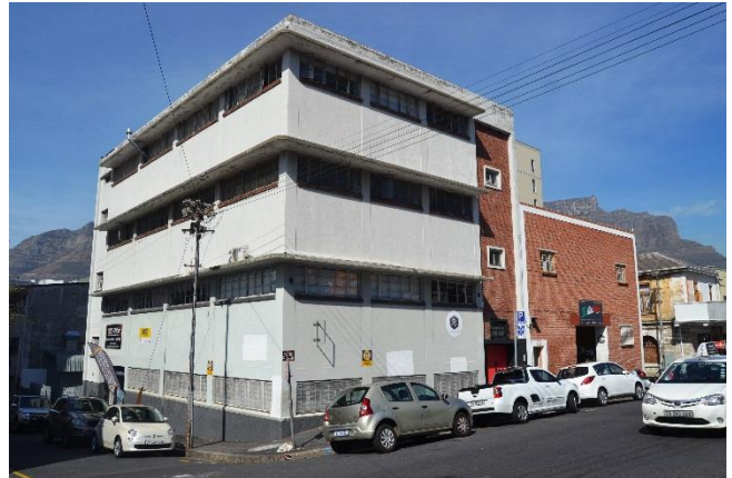
View 2: Looking east across Rose Street
