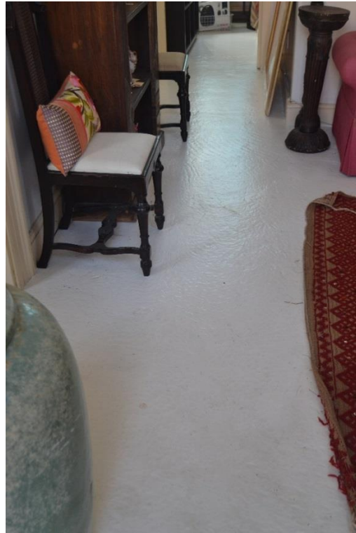
View 2: Painted concrete floors
