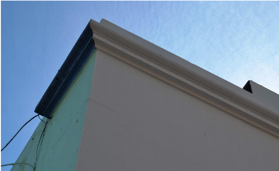
Rose Street façade parapet moulding
