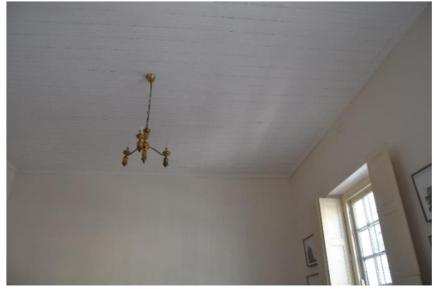
View 6: Living room ceiling
