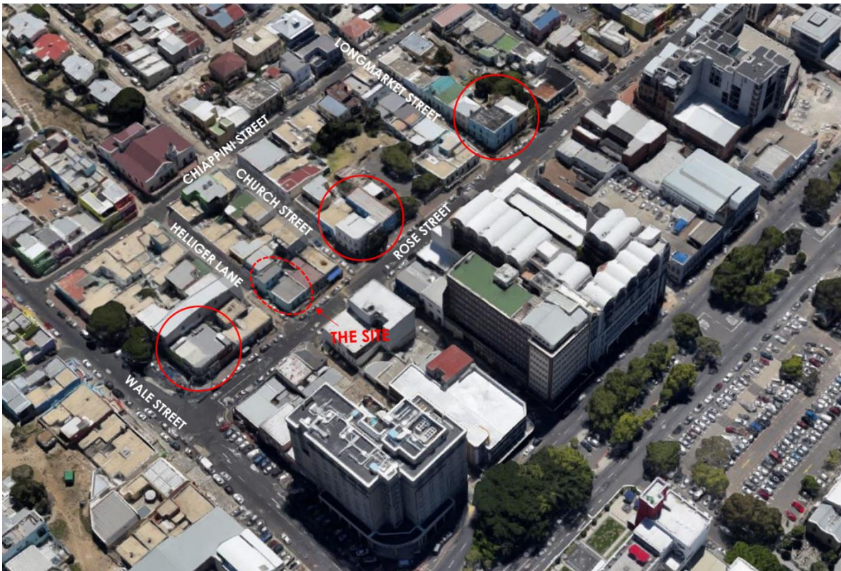
Three corner block two storey buildings on Rose Street near to the site
