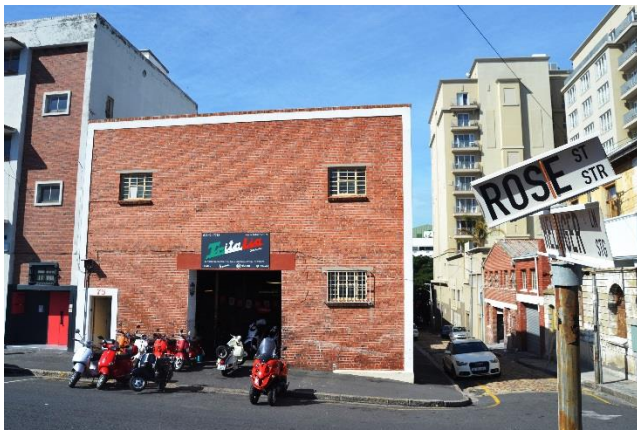
View 3: Looking directly across Rose Street
