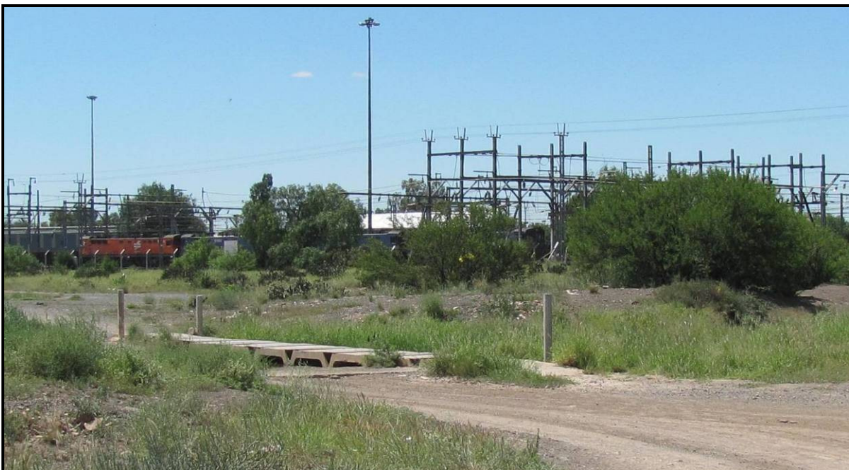
Plate 1: Proposed location for retention dam 1 - view eastward toward the railway lines.
