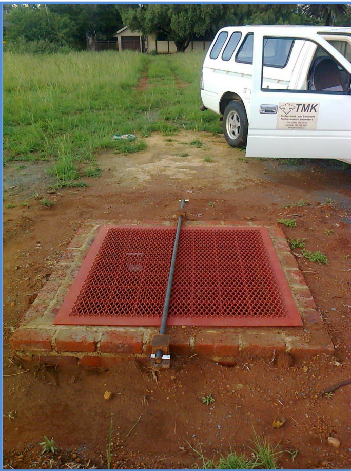
Plate 4: View of borehole equipment
