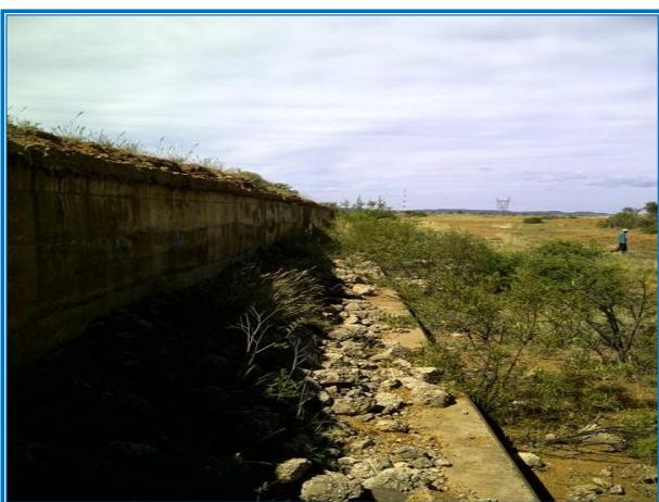
Plate 15: Another view of decommissioned SANDF site
