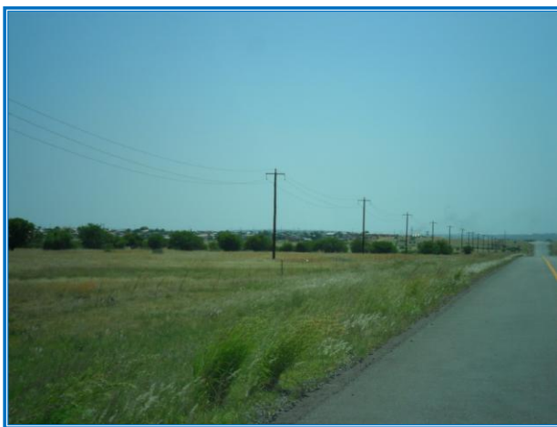
Plate 25: View of Eskom Leeufontein Rural / Trotsville 1 (22kV) Feeder MV Overhead Line along Road N12
