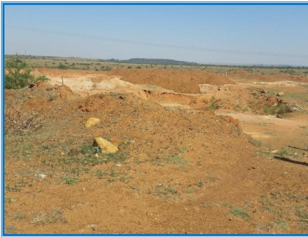
Plate 8: View of quarry / excavation area
