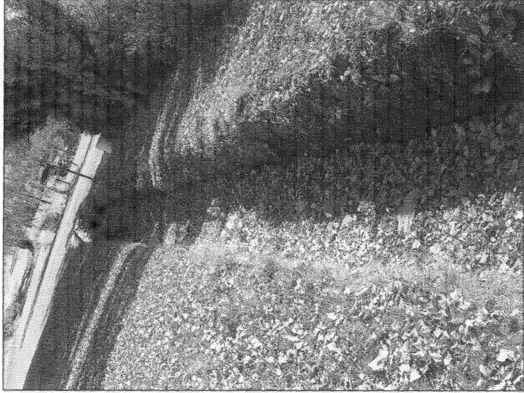
Fig.23 Sand stone kerb and storm water ditch in Vorster Street.
