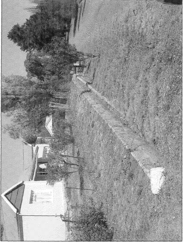
Fig.21 Sand stone storm water furrow in Muller Street.
