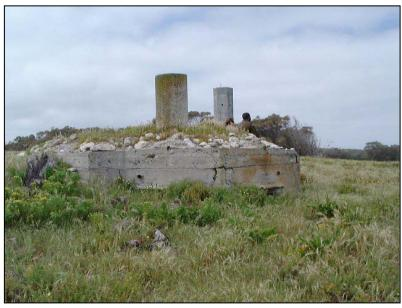
**DESCRIPTION:** hexagonal 3 story high concrete observation tower indicated by Riley to be a radar position. Nearby a portion of machinery (?radar mounting) lies on the ground in long grass. Observation ports have been covered over with wood perspex. and There is no evidence of heavy steel shutters characteristic of WW2 period buildings. Access between the floors is via steel The ladders. ground floor of the tower has plastic tiles on the floor and contains a toilet.
