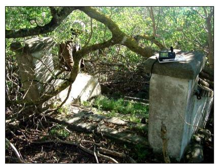
DESCRIPTION: A cast concrete machine gun post with its 3 gun ports directed over the central golf course area of the island. There is a rear entrance hatch with a steel cover, interior is in good order.
