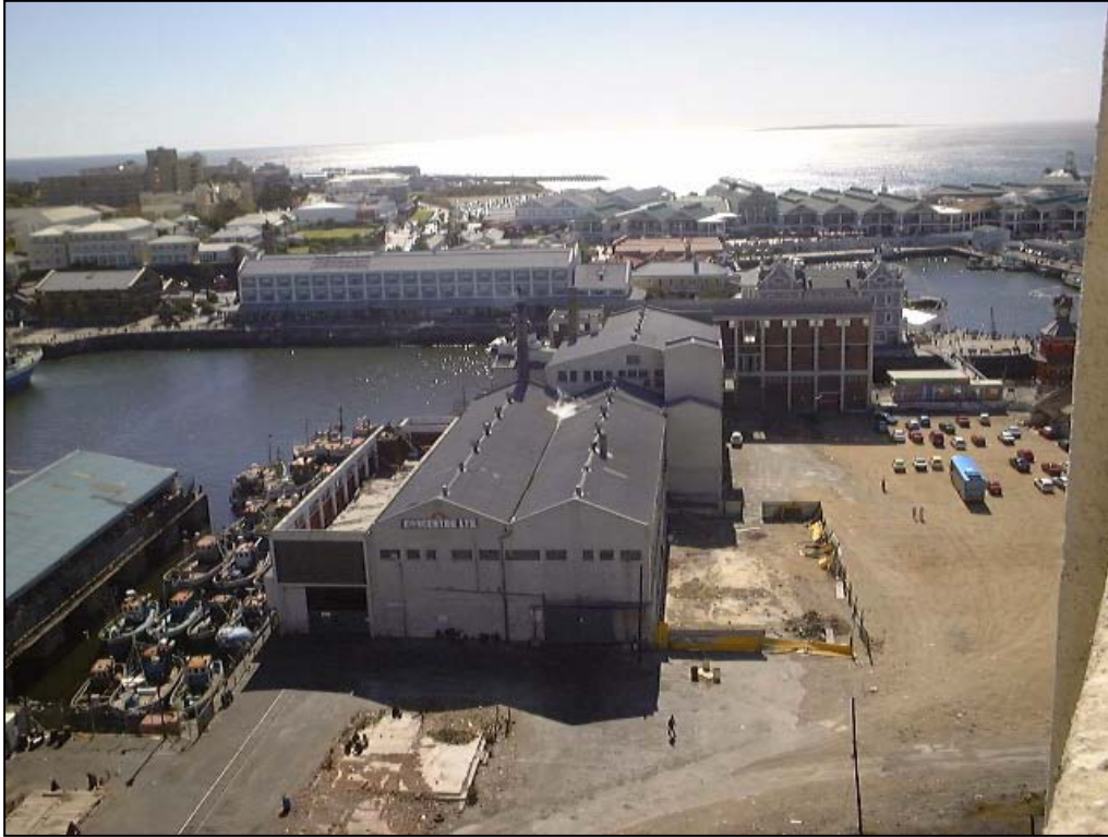
Figure 8 The Concentra Factory over the site of the Chavonnes Battery in January 1999 prior to demolition.
