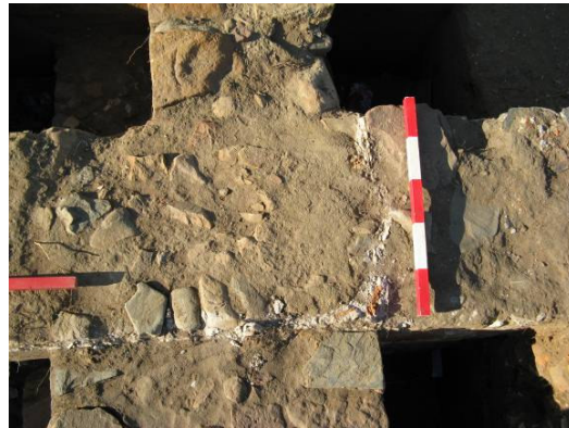
Plate 4: The plaster line showing the exterior corner of the original core.
