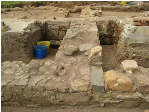
Plate 3: The construction method used in the stoep is similar to that used in the original core, but with a brown clay mortar. NW corner.
