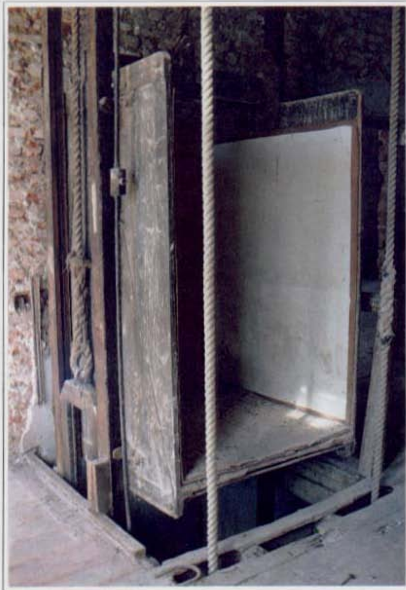
PLATE 8: View of the simple rope operated lift.
