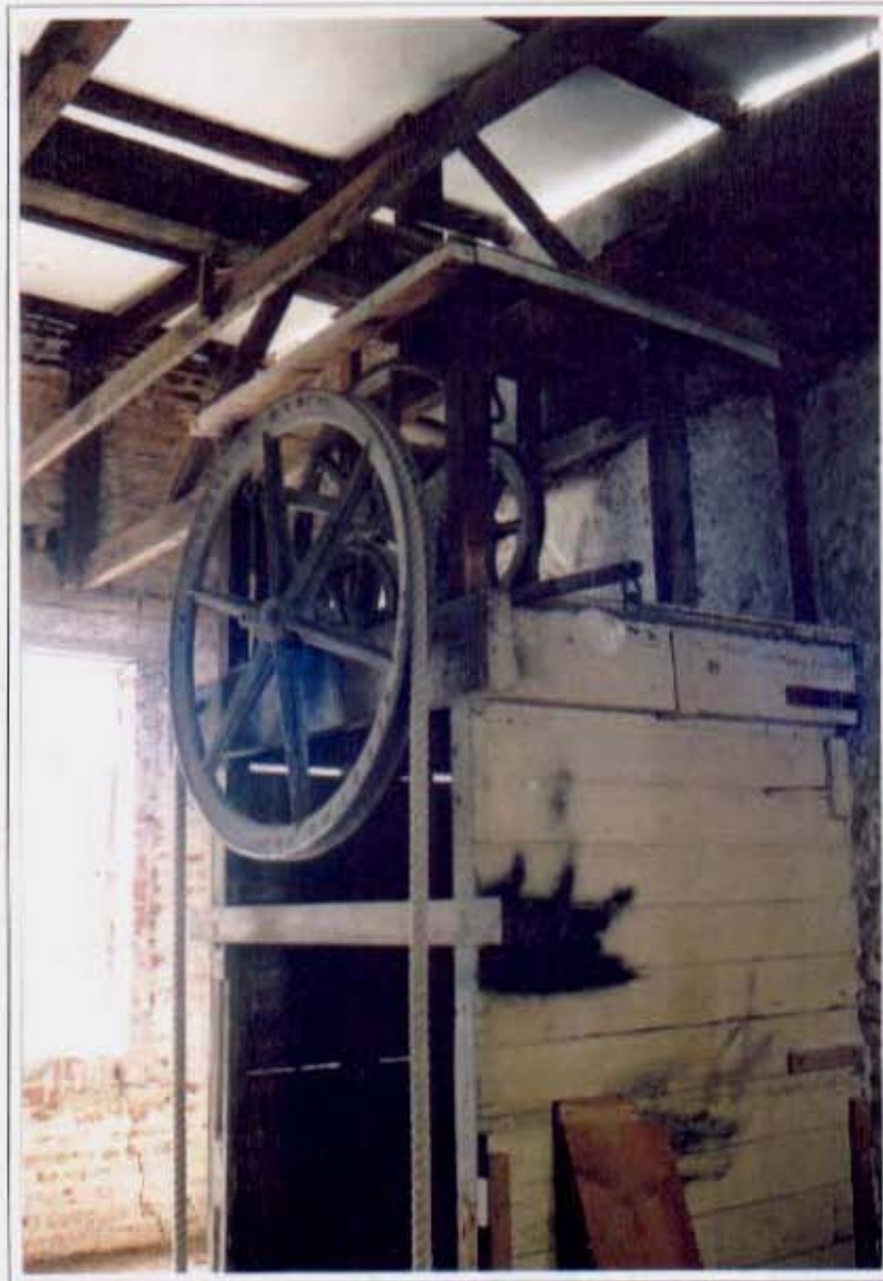
PLATE 9: Winding mechanism of the rope operated lift which is still in working order.
