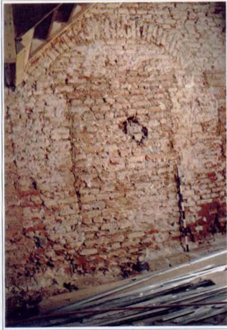
PLATE 3: One of three bricked up 18th century openings with relieving arches.
