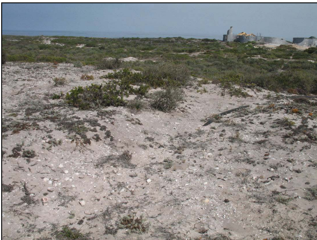
Figure 8: The water pipe in place at Point H. Although shell was disturbed during the trenching for this pipe, the material at the surface suggests that no dense shell midden is located within the uppermost 20 to 30 cm.
