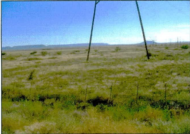
Figure 11. North West Option powerline servitude facing east
