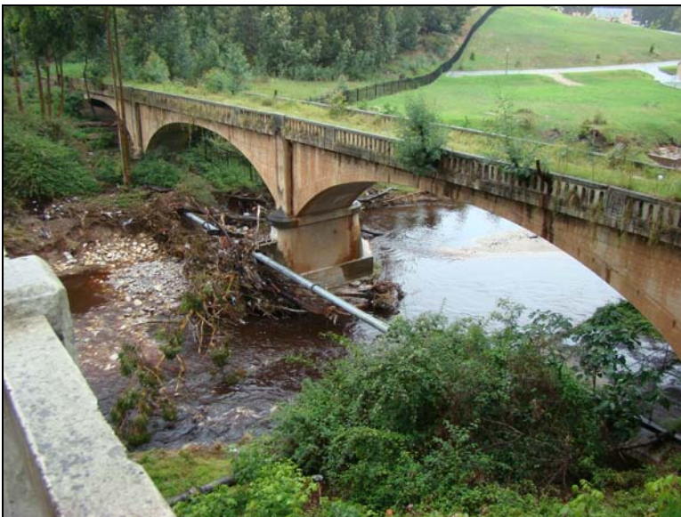
Fig.12 Point 17 at the bridge crossing the Malgas River.
