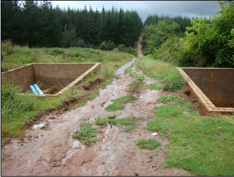
Fig.1 Point 1. Starting point of the Blanco water pipeline.
