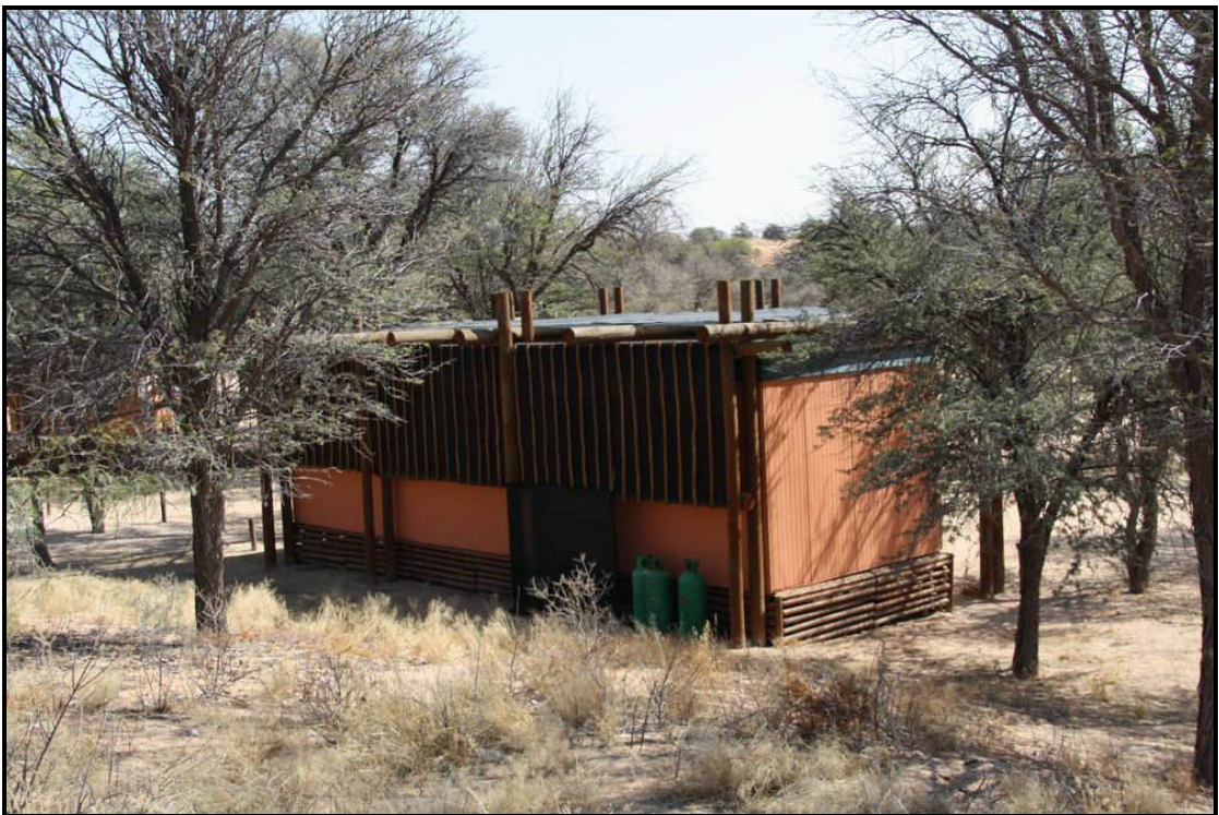
Fig. 8 & 9. Front and rear view of one of the parkhomes.
