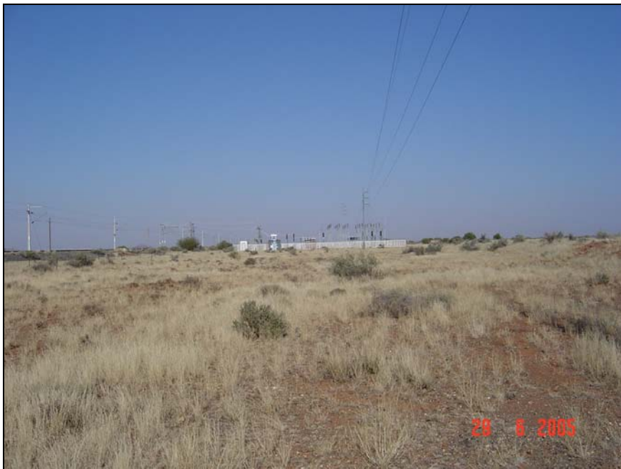
Fig.1 Wigton Substation. Ballast banking of the old railway line is visible on the right.
