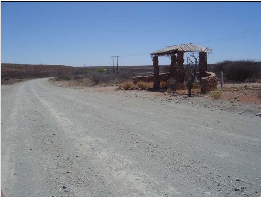
Fig.14 (7) Position of the power line on the border of Naauwtesfontein 78 & Disselfontein 77 along the way to the Disselfontein Substation
