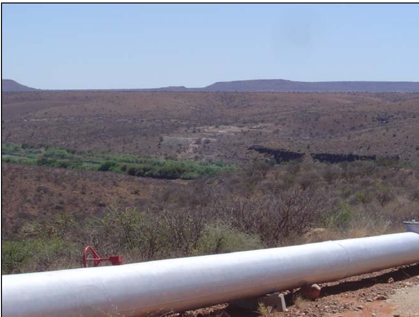
Fig.12 View towards the Orange River. The power line will cross at the high cliffs in the centre right of the picture.
