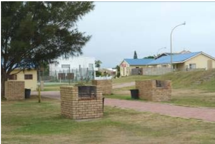
Fig. 5. An example of the buildings and other structures.
