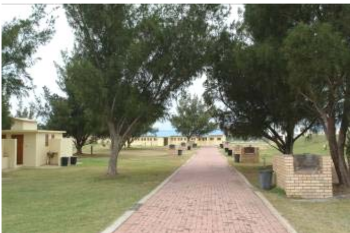
Fig. 6. Brick paved roads and grass covered top soil.
