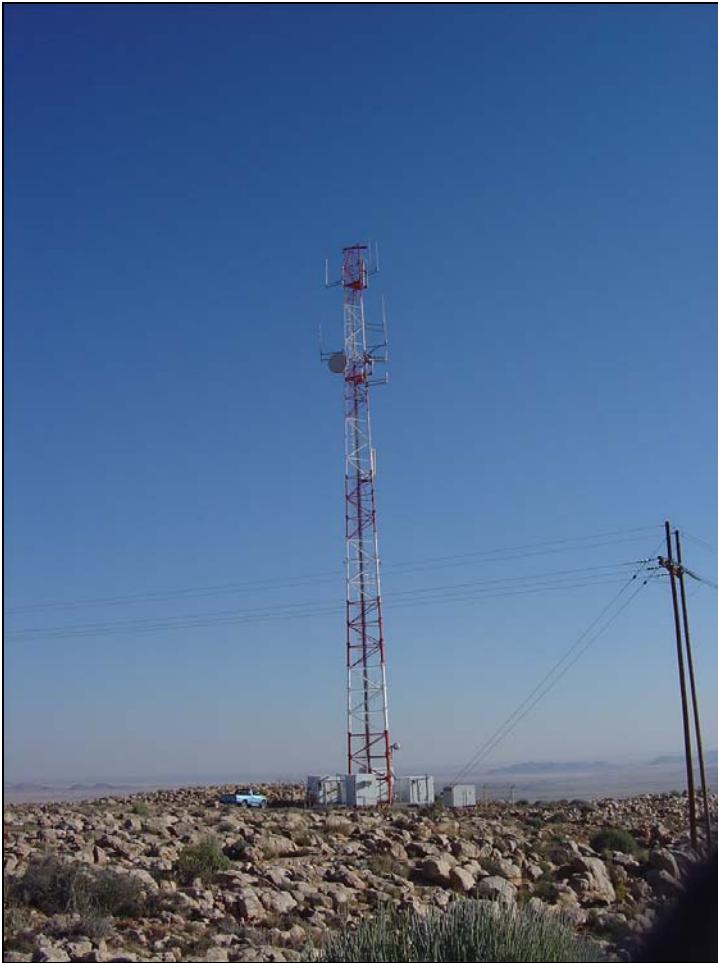
Fig.4 Full view of the Gamsberg lattice mast.
