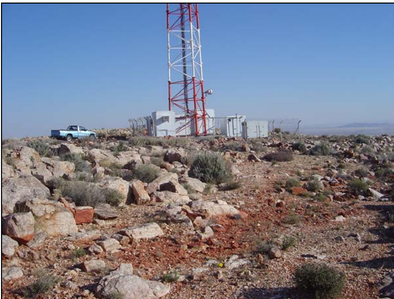
Fig.3 View of the lattice mast and its surroundings on the mountain.
