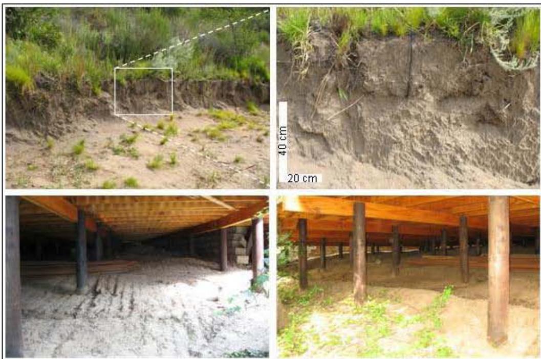
Plate 4. Top - exposed profile on edge of " fire break" (red dot above "d" in Figure 5) and - bottom - exposed ground under new structure show sandy surface sediments typical of the study area.
