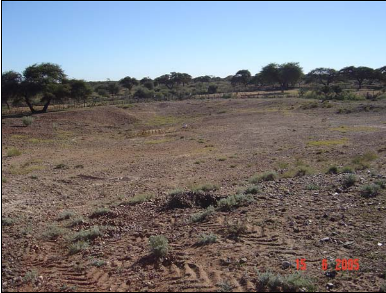
Fig.9 Borrow Pit 3 (Existing borrow pit).
