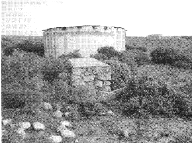
Figure 10. Concrete dam and block.
