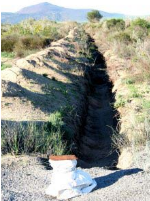
Figure 5. Capped borehole at the beginning of the metre deep, kilometre long trench next to the proposed route.
