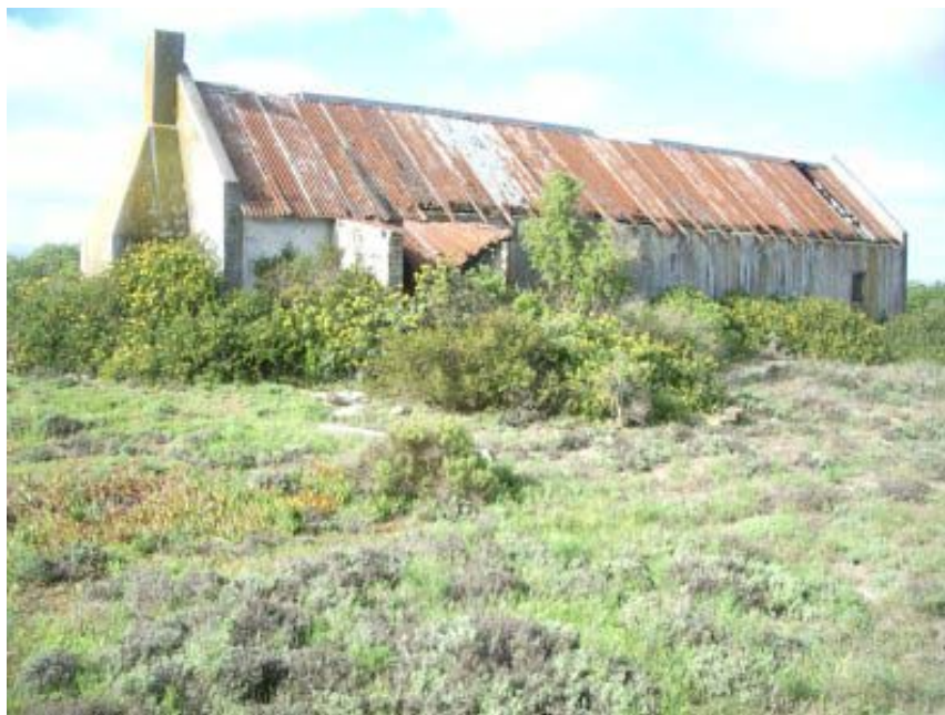
Figure 11. Ruined building in the southern portion of the property. GPs reading S° 33 24 000 E 18° 13 717.
