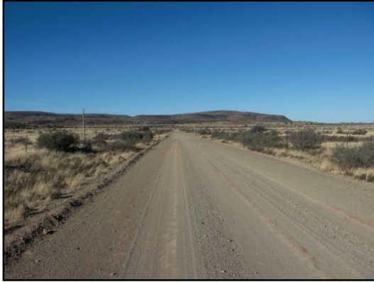
Figure 53: General view of the road surface and reserve: DR2631
