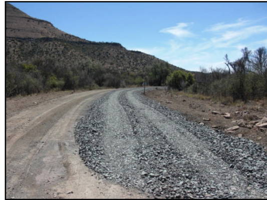
Figure 40: Upgrading of Road nr 654 in progress
