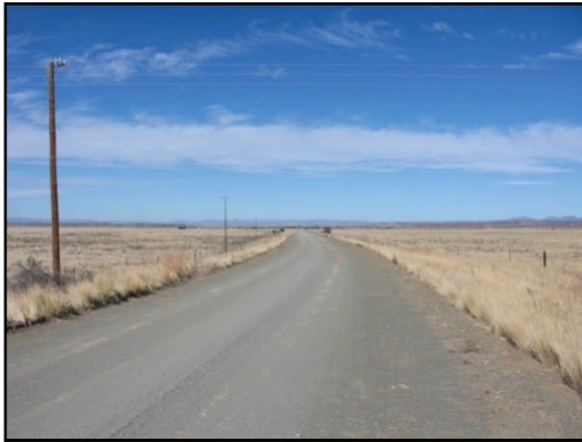
Figure 39: Road nr 654 - General view of the gravel road surface
