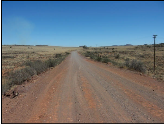
Figure 4: General view of the DR2629
