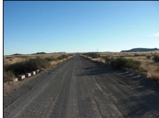
Figure 54: General view of the DR2631
