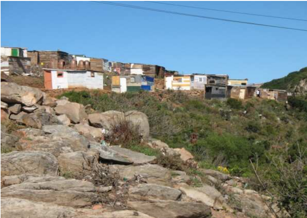
Plate 14. The north-eastern corner of Zinyoka informal settlement
