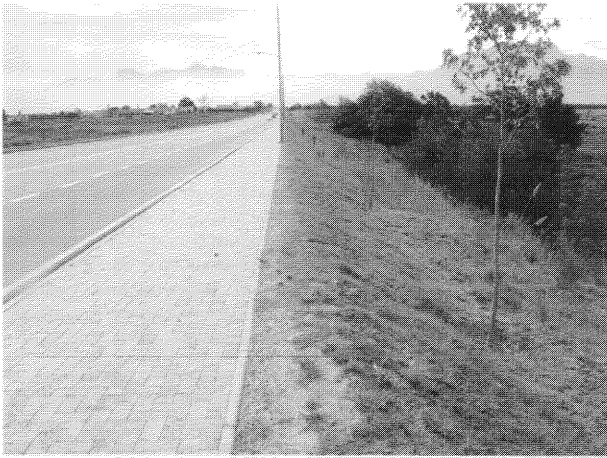
Figure 3. Beach Road, Pacaltsdorp
