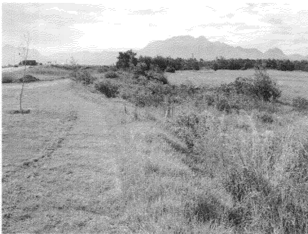
Figure 4. Beach Road, Pacaltsdorp
