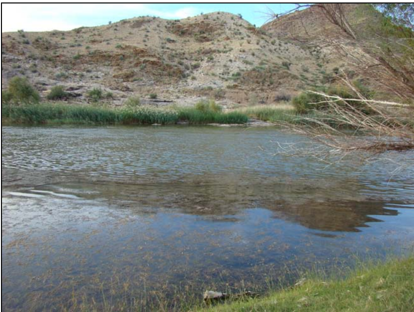
Fig.4 Weir site at Blouputs, Northern Cape.
