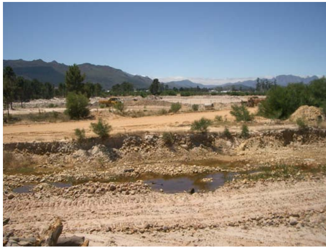
Figure 8. The site facing north west.
