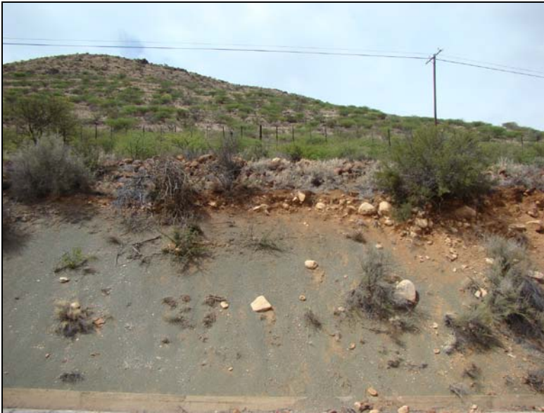
Fig.16 Point J in the cutting along the pipe line route outside Vanderkloof.
