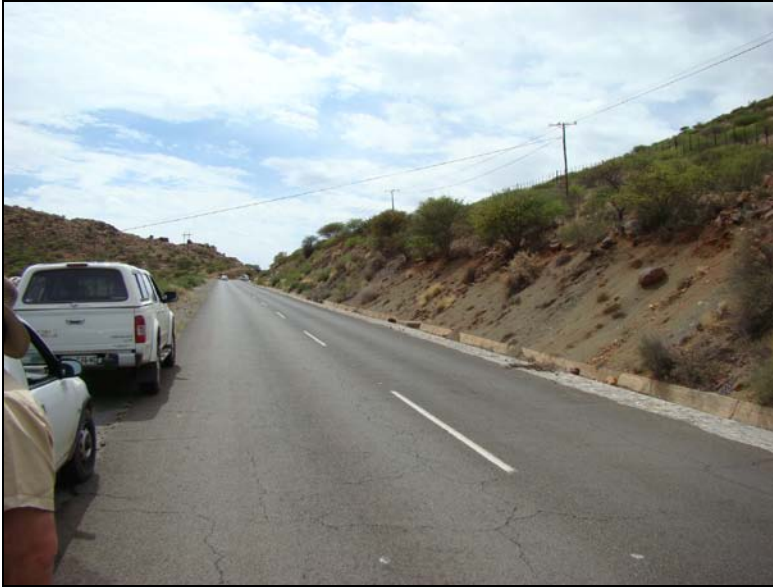
Fig.18 Point J in the cutting along the pipe line route outside Vanderkloof.
