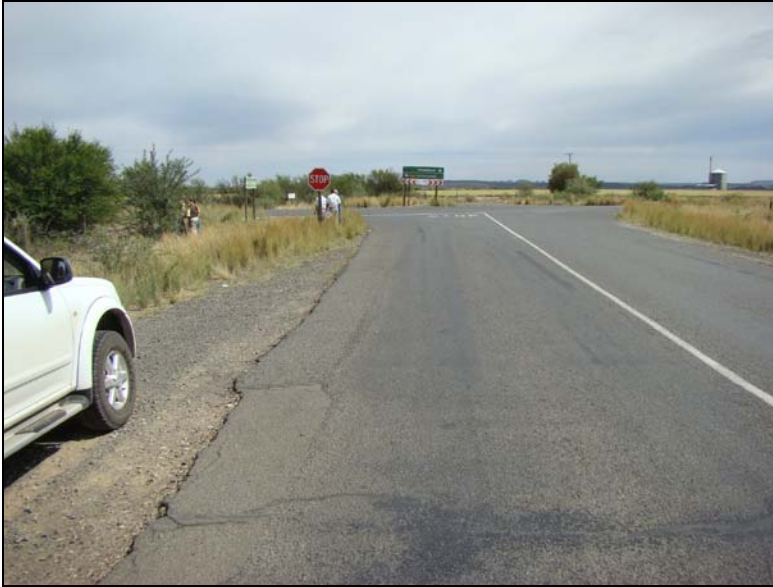
Fig.10 Point F along the pipe line route from Vanderkloof to Petrusville.
