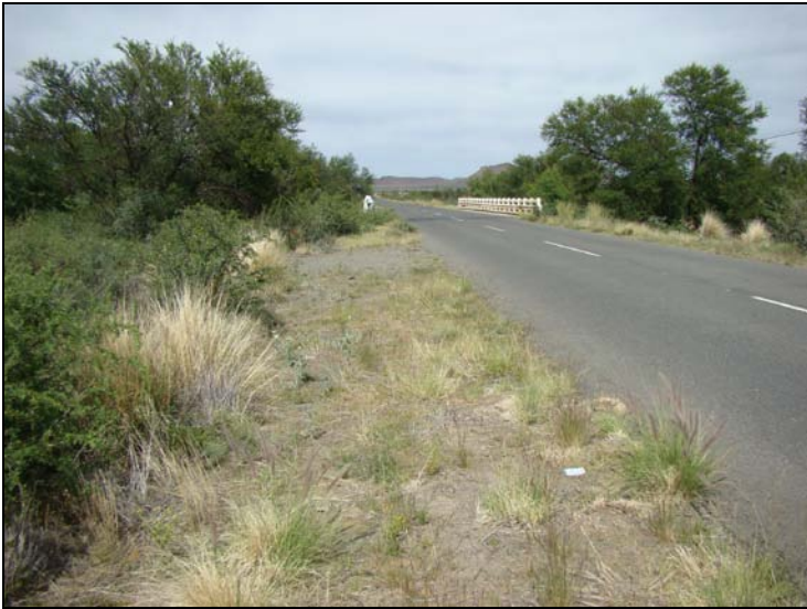
Fig.12 Point G along the pipe line route from Vanderkloof to Petrusville.
