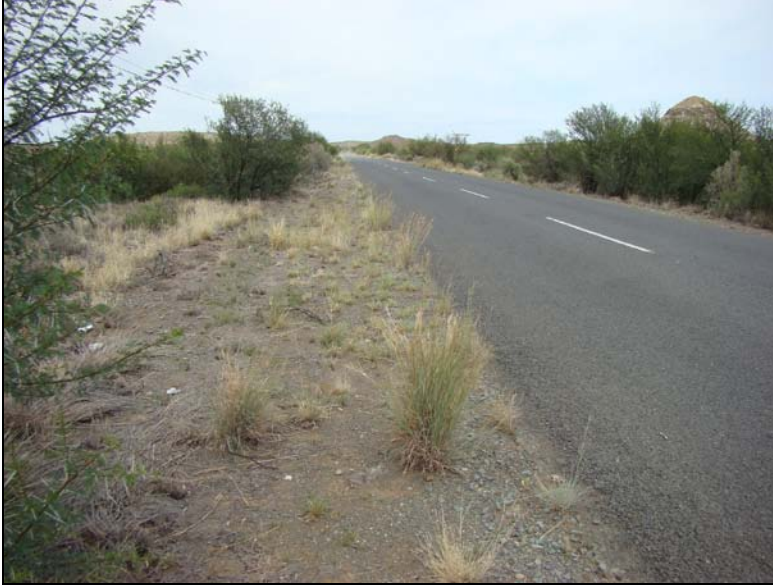
Fig.14 Point H along the pipe line route from Vanderkloof to Petrusville..
