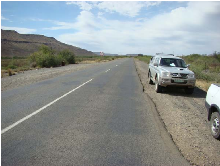
Fig.9 Point F along the pipe line route from Vanderkloof to Petrusville..
