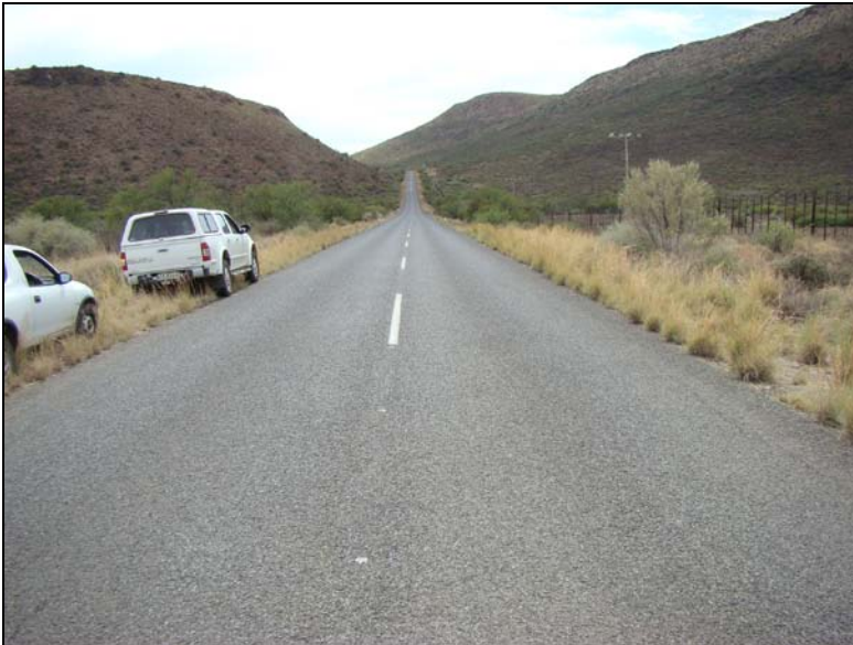
Fig.15 Point H along the pipe line route from Vanderkloof to Petrusville.
