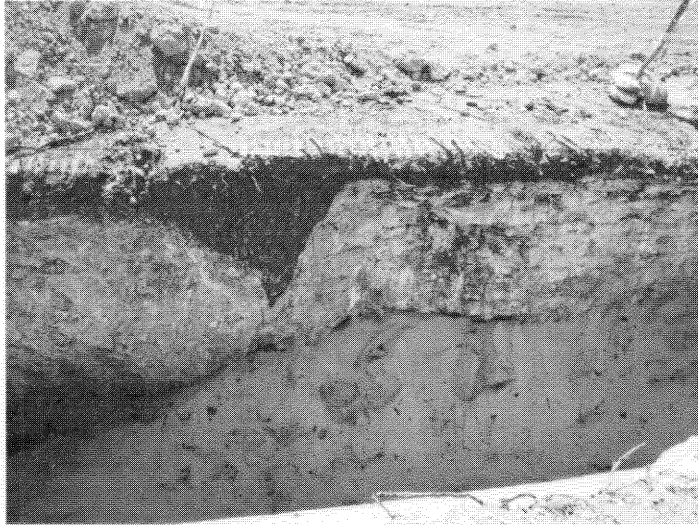
Fig. 2: A trench for a pipeline showing the red-brown topsoil, a thin scattering of quartzite cobbles, and the lower calcrete deposits.
