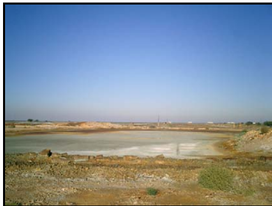
IMAGE 16: Partial view over the drying pans / pyrite slabs (P)
