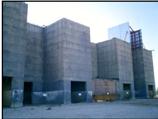
IMAGE 14: General view – the crusher plant (back)
