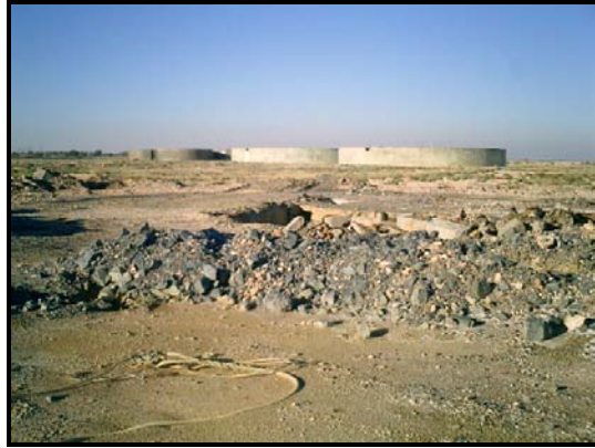
IMAGE 12: Cemented plant platform with cyanide dams
