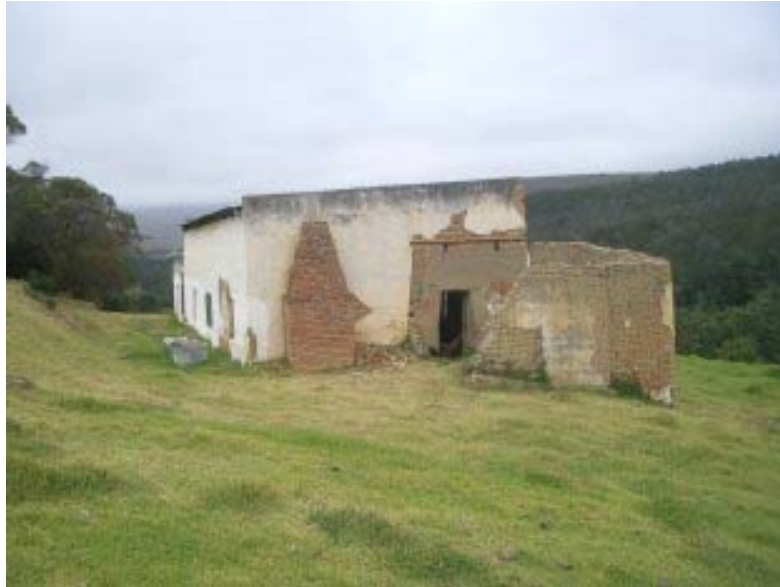
Figure 6. Ruined building on the farm (view from the north side).
