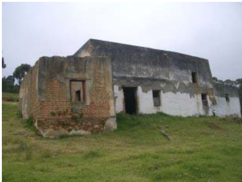
Figure 7. Ruined building on the farm (view from the front).
