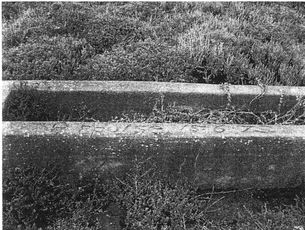
Figure 14: Water trough in front of building. Signed and dated A. Paulse 15.6.73.
