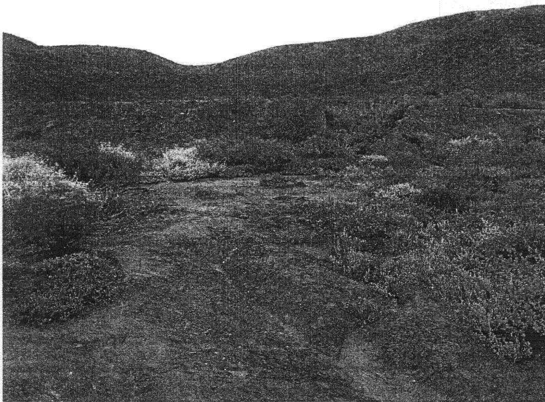
Figure 10: Breached earth dam and resultant erosion.
