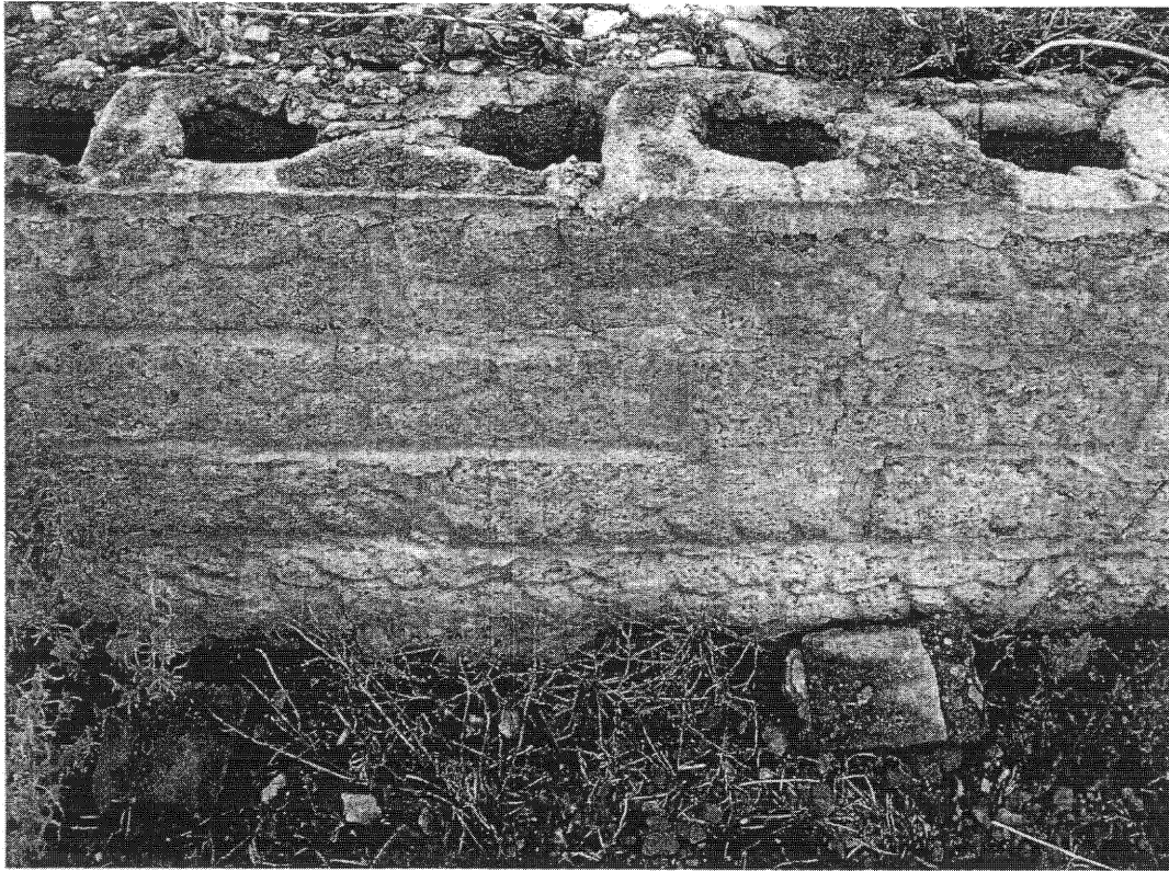
Figure 9: Detail of building. Note the patterned breeze-block construction typical of the 1960's and 1970's.
