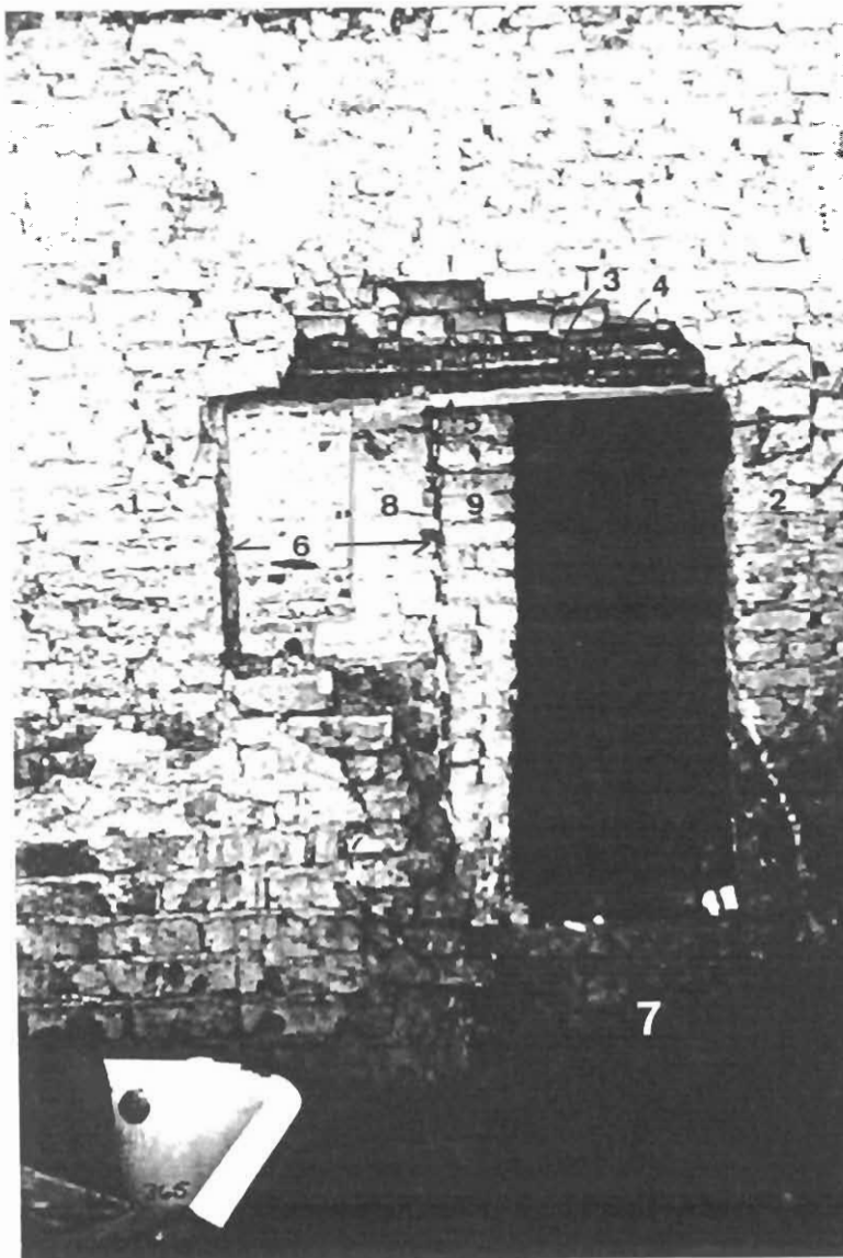
36.1 A similar view of Room D2 as photo 36. Note that the raw brick on either side (1 & 2), line perfectly up at the reveals (c.1735). There are two lintels (3 & 4). The door was diminished (lintel painted white)(5), with a window (6) adjacent to it during the 19 th century. They were both blocked-up by the late 19 th century. In Room E, a remnant of the old hearth base in brick and wall above (8), later received an arched doorway (>1900). Wall A1 represents the pantry wall of c.1860 (9). (looking E)(Le Roux 1974).
