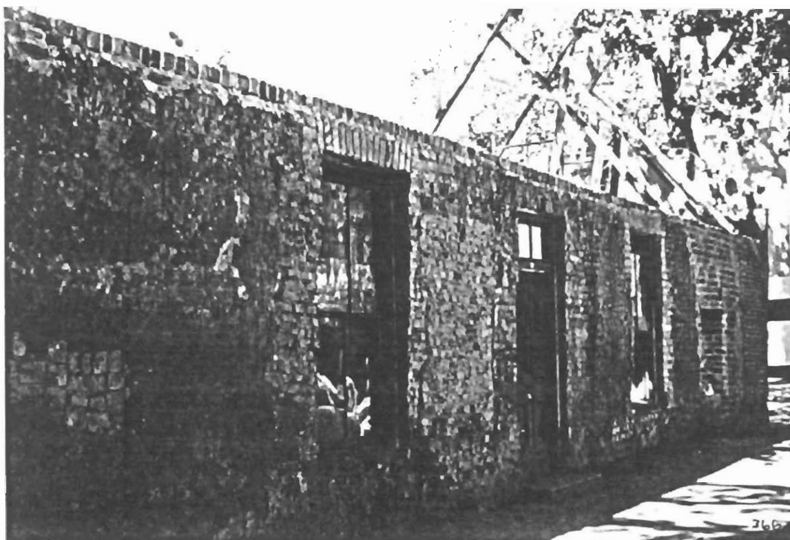
4. View of the façade, prior to most of the 1975 alterations. Note how little is even left of the >1730 raw brick walls. Much patching in 19 th century brick is obvious (Le Roux 1974).
