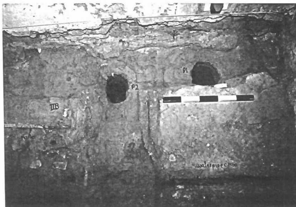
52. Same view of the post-holes (probably dug for scaffolding posts), both post-dating 1840. A piece lead lie above P1 in an upper layer. Hearth IIB is visible on the left.
