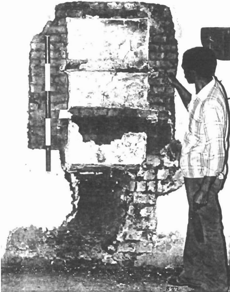
18. A small cupboard was cut into wall D2 and the filled-in brick was carefully removed to reveal its construction (>1740).
