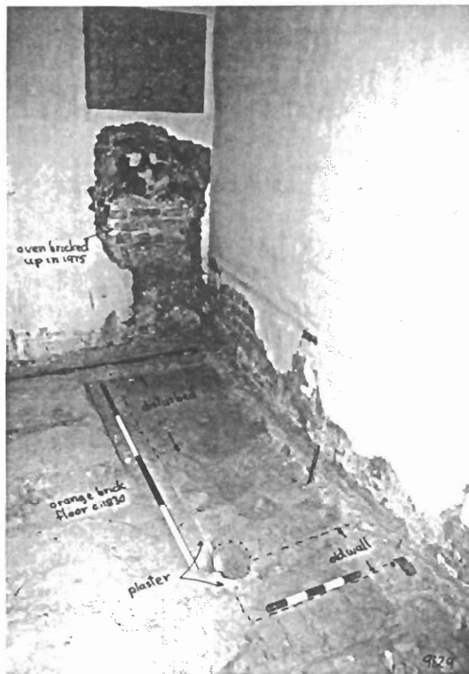
30. In 2000 the old oven opening was partially exposed to determine its exact position in relation to the raised hearth.
