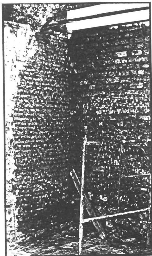
27. View towards the corner AA4/2, to show the contrast. Left (AA4): flat raw brick above a low (20-30cm) stone foundation. Right (AA1): A 50cm undressed stone foundation with hard-fired orange brickwork of the late 18 th century (Le Roux 1974).
