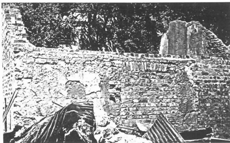
13. Tail end, exterior (E1) with clayed-up walls on left (looking S) (Le Roux 1975).
