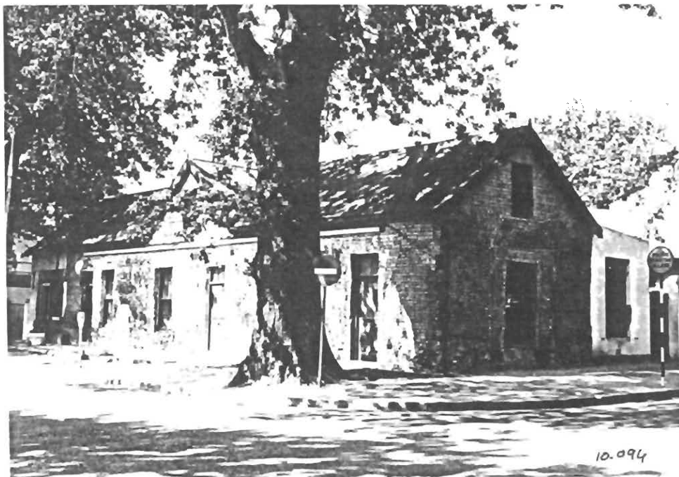
FIG.45.2 View of Schreuderhuis after the plaster was stripped in 1973 (Studio 7, Johan Stander; SB Museum).
