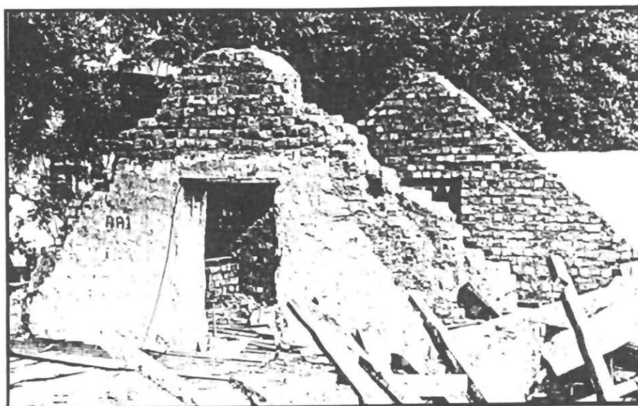
27. View towards the corner AA4/2, to show the contrast. Left (AA4): flat raw brick above a low (20-30cm) stone foundation. Right (AA1): A 50cm undressed stone foundation with hard-fired orange brickwork of the late 18 th century (Le Roux 1974).
