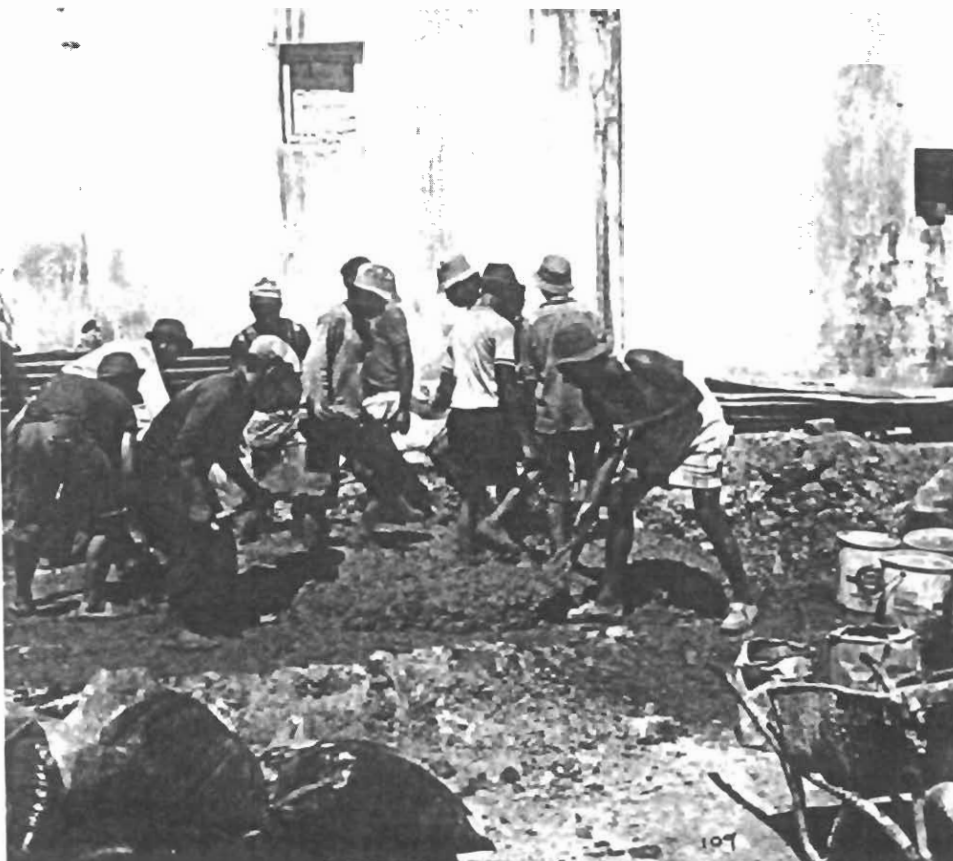
62. Men trampling the clay before it was cast as the clay floor for Schreuderhuis in 1975. Site was just behind SH with Berghhuis at the back (Vos 1975).
