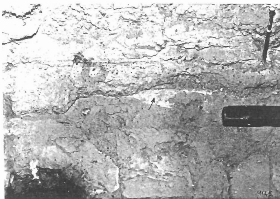
39. In Room E, against wall B4 (unit B), underneath the yellow clay, remnants of limewash may indicate that the orange brick floor was once limewashed. The one post-hole is partially visible on the left.
