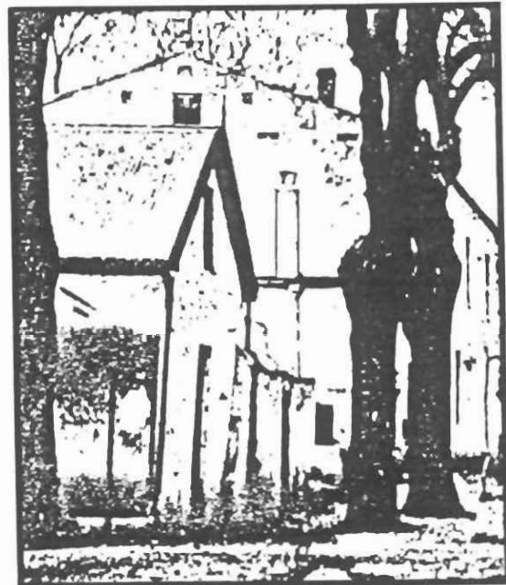
FIG.38 View of Schreuderhuis with the boundary walls along Church Street (c.1930)(SB Museum).
