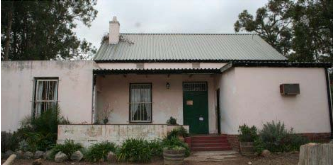
Figure 9. Building C, original house probably early 1900s, much modified with afdaks.
