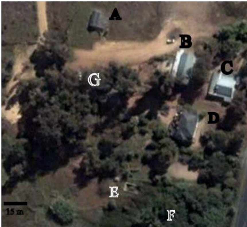
Figure 4. Buildings A-D, G avenue of trees, E derelict swimming pool, F spring.
