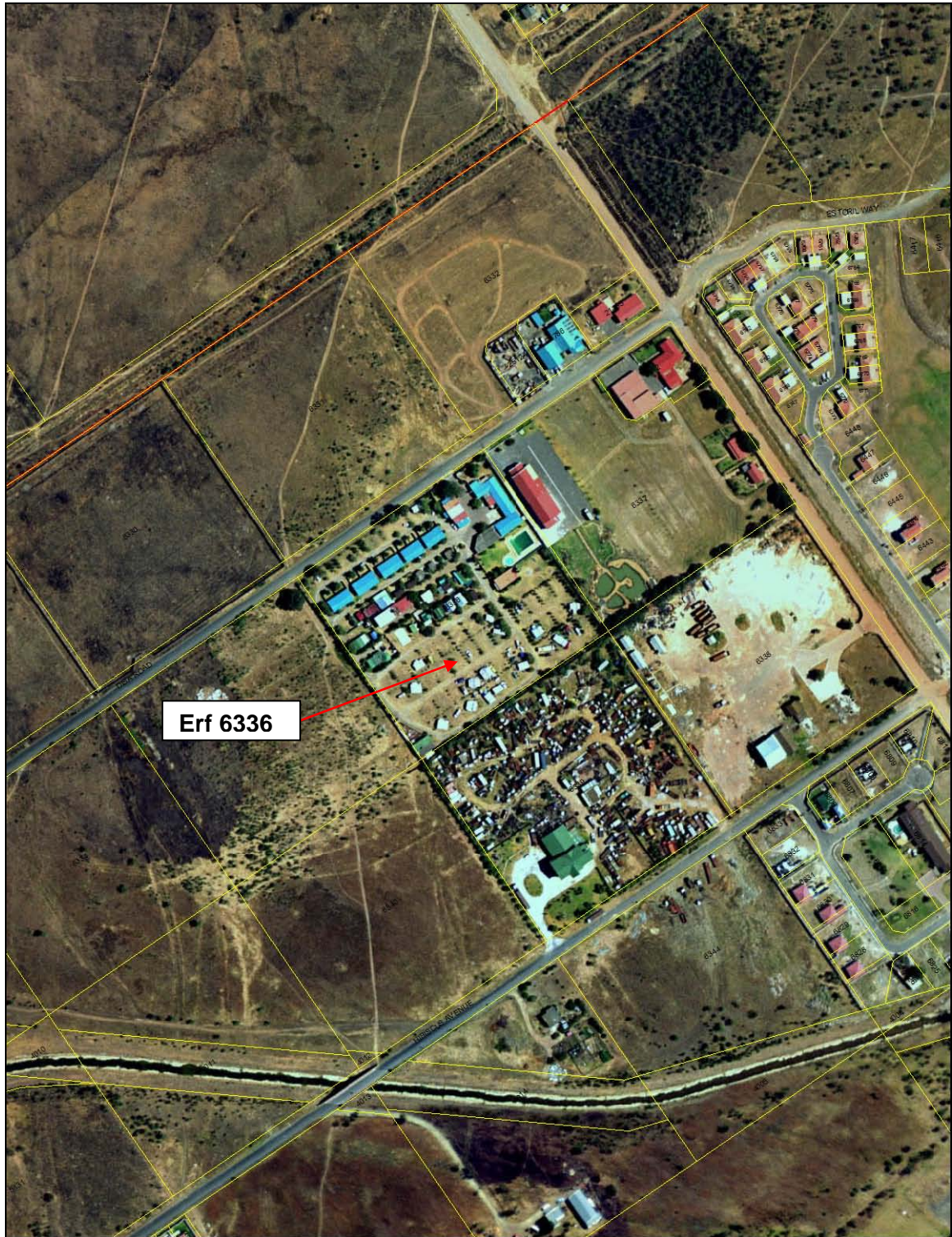
Figure 2. Aerial photograph of the site.
