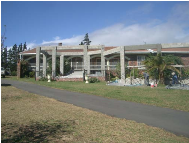
Figure 10. Main house under renovation.
