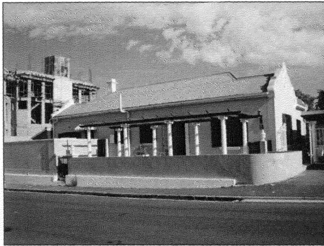
Fig. 17a. The street façade, 18 Hill Street, 2007. Note the back of the house faces the street. The stoep is cemented over. To the left an enclosed yard, accessed from the kitchen. No front garden was retained.
